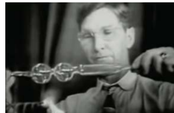
SCIENTIFIC GLASS-BLOWING PROCESS John Lehman - Master Glass Blower 1951
