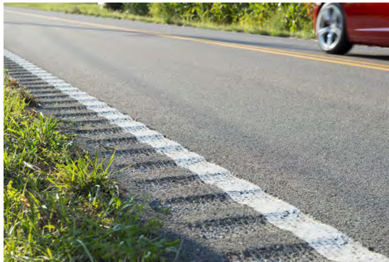
Figure 2.19: A visual shows road rumble strips.
